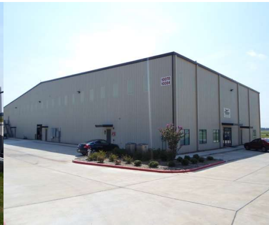
Entrance to Office Area
