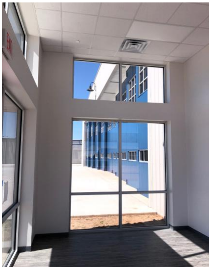
Hangar 6-A Lobby View
